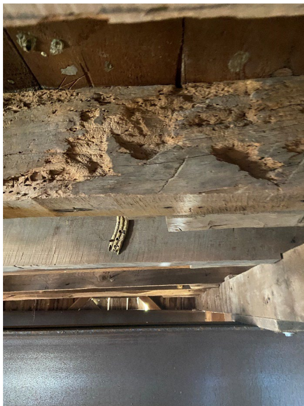
Photo 10 – Deteriorated joist.
