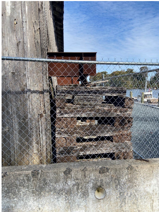
Photo 2 – Deteriorated cribbing.
