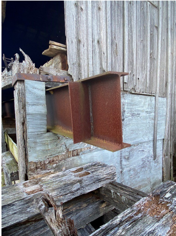
Photo 3 – Deteriorated cribbing.
